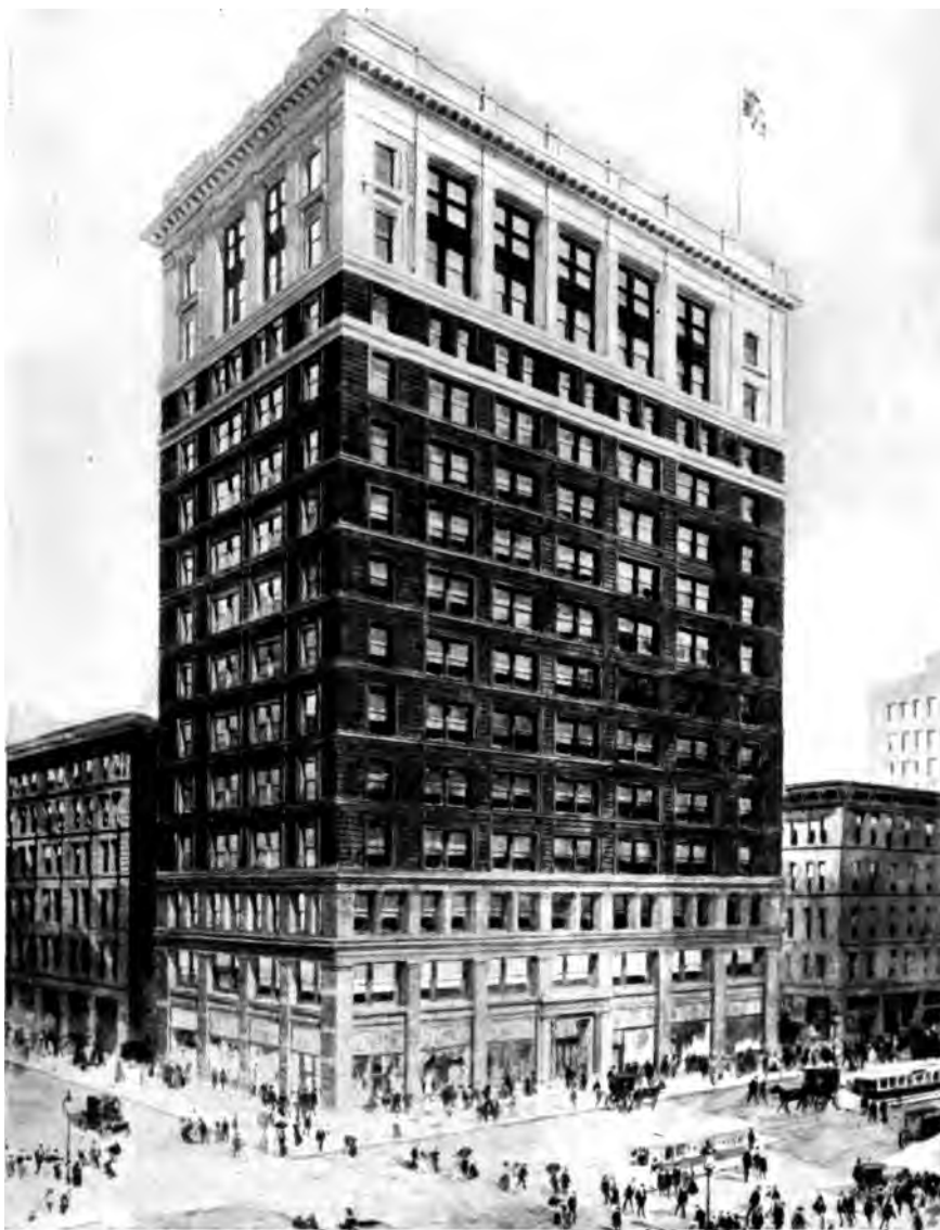
THE TRACTION BUILDING, Cincinnati, Ohio.
